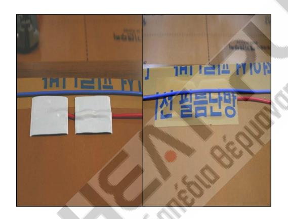
7. Insulating the soldered area with a butyl tape
